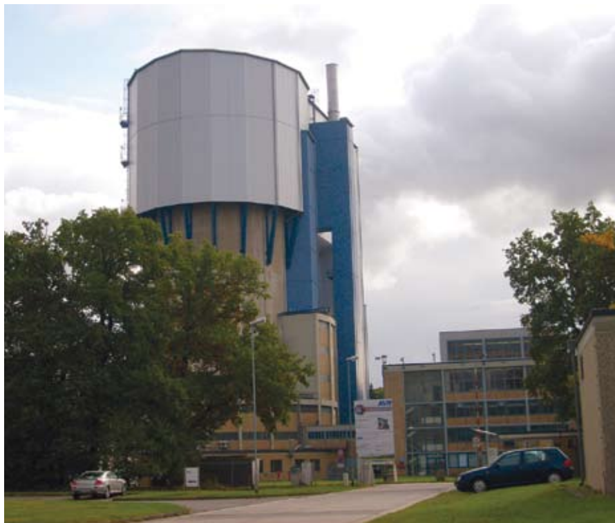
The AVR experimental high temperature reactor. Dr. Cleve headed the engineering team that designed and built the nuclear reactor.
