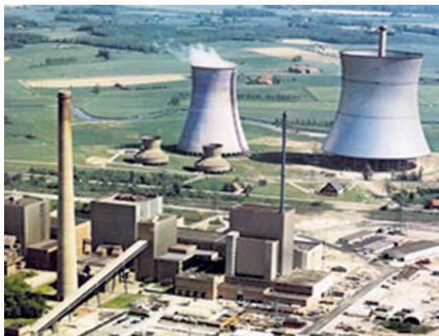
The successor to the AVR: The 300-megawatt Thorium High Temperature Reactor (THTR) operated for three years, until it was shut down for political, not technical, reasons.
