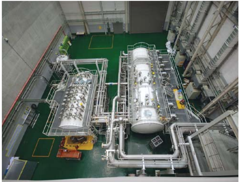
The KSTAR cryogenics system used to cool down the superconducting magnets.
