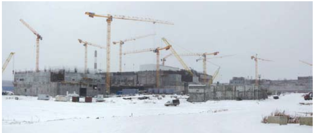
Russia's BN-800 fast reactor in construction.
