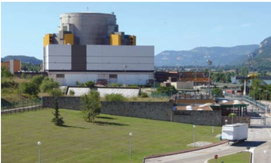
The largest fast breeder reactor was built in France, the 1,200-megawatt-electric Superphénix. It was shut down in 1998, for political reasons.
