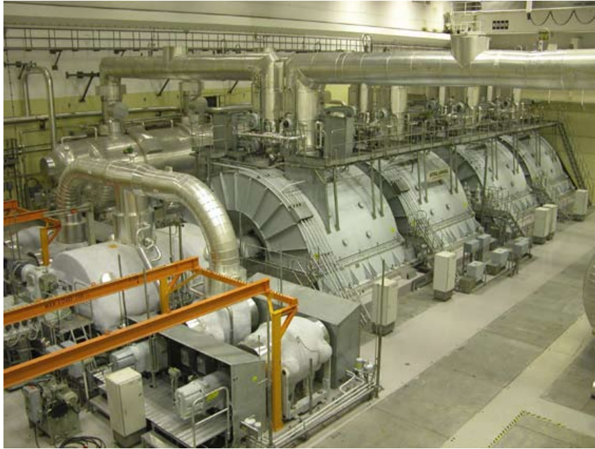
Steam turbine at TVO's Olkiluoto nuclear power plant in Finland. Olkiluoto is a Swedish-built boiling water nuclear reactor, where steam goes directly from the reactor to the turbine.
