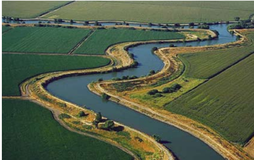
California Department of Water Resources
