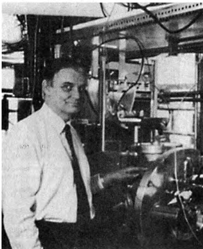
*Paul Marmet, shown with the electron spectrometer that he pioneered, at the Herzberg Institute of Astrophysics. The spectrometer produces a low-energy, monoenergetic electron beam, which is used to study aspects of the electron structure of atoms and molecules, such as their energy levels.*
