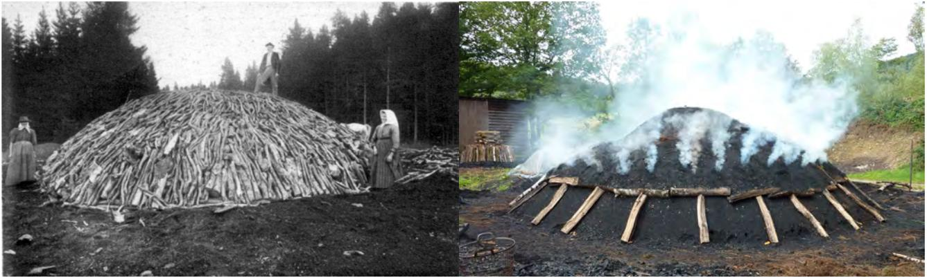
*Charcoal production: a century ago, and as recreated in modern times. The production of charcoal represented an important transformation. Wood, which contains many different chemical substances, is stacked in a large pile, covered with soil, and burned slowly in an oxygen-poor environment for a few days. The resulting product, charcoal, is almost entirely pure carbon. Charcoal is highly porous, allowing greater airflow in a furnace, and therefore higher temperatures and more rapid heating.*
